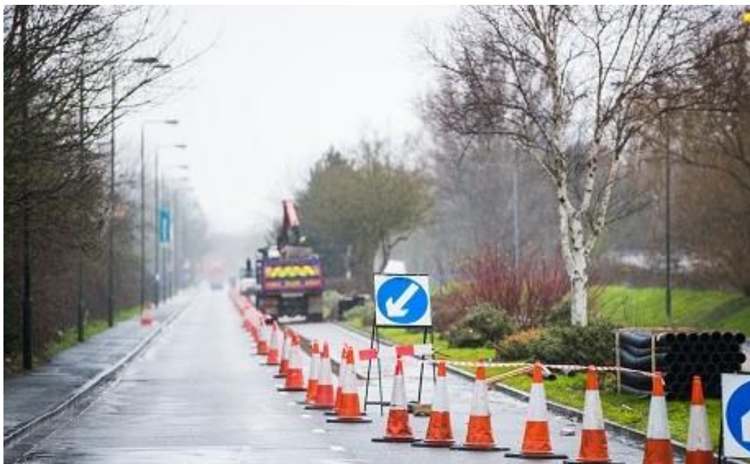
Plate 3.18: Example approach to cable working area
