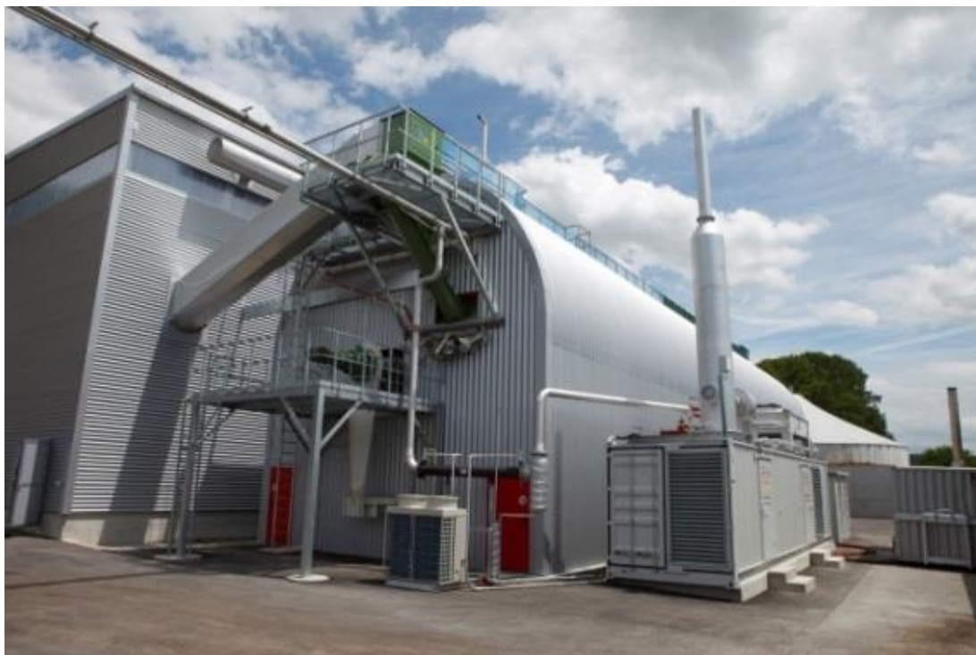
Plate 3.13: Example digester
